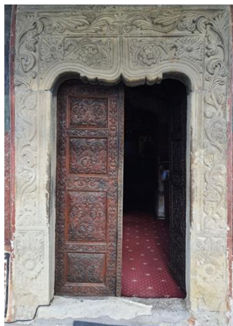
Figure 9. Framing of the entrance door - stone sculpture at Govora Monastery.
